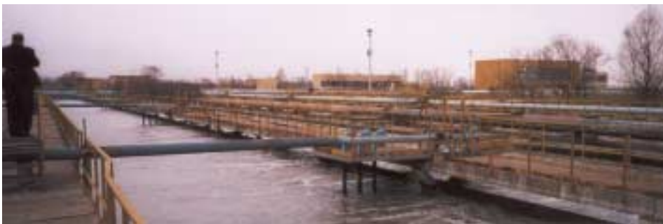
Alan Will inspects one of the Sofia WWTP aeration basins
